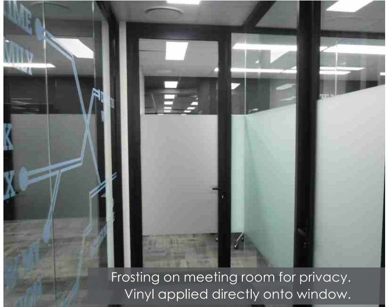
Frosting with Vinyl applied over the top.
